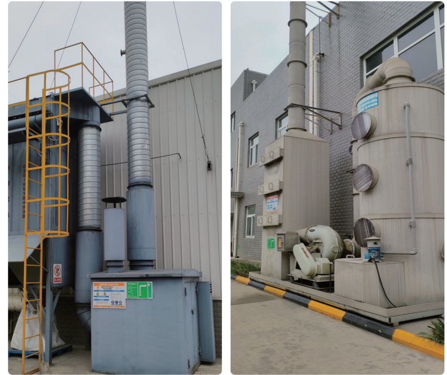
Silicon carbide dust control equipment and Exhaust gas treatment systems
