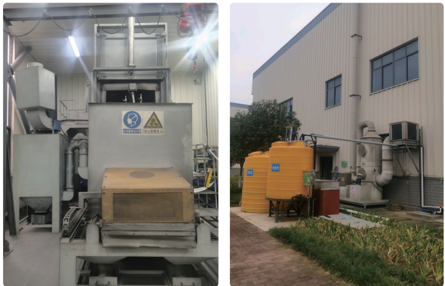
Shot blasting dust collection system and Acid wash wastewater treatment equipment
